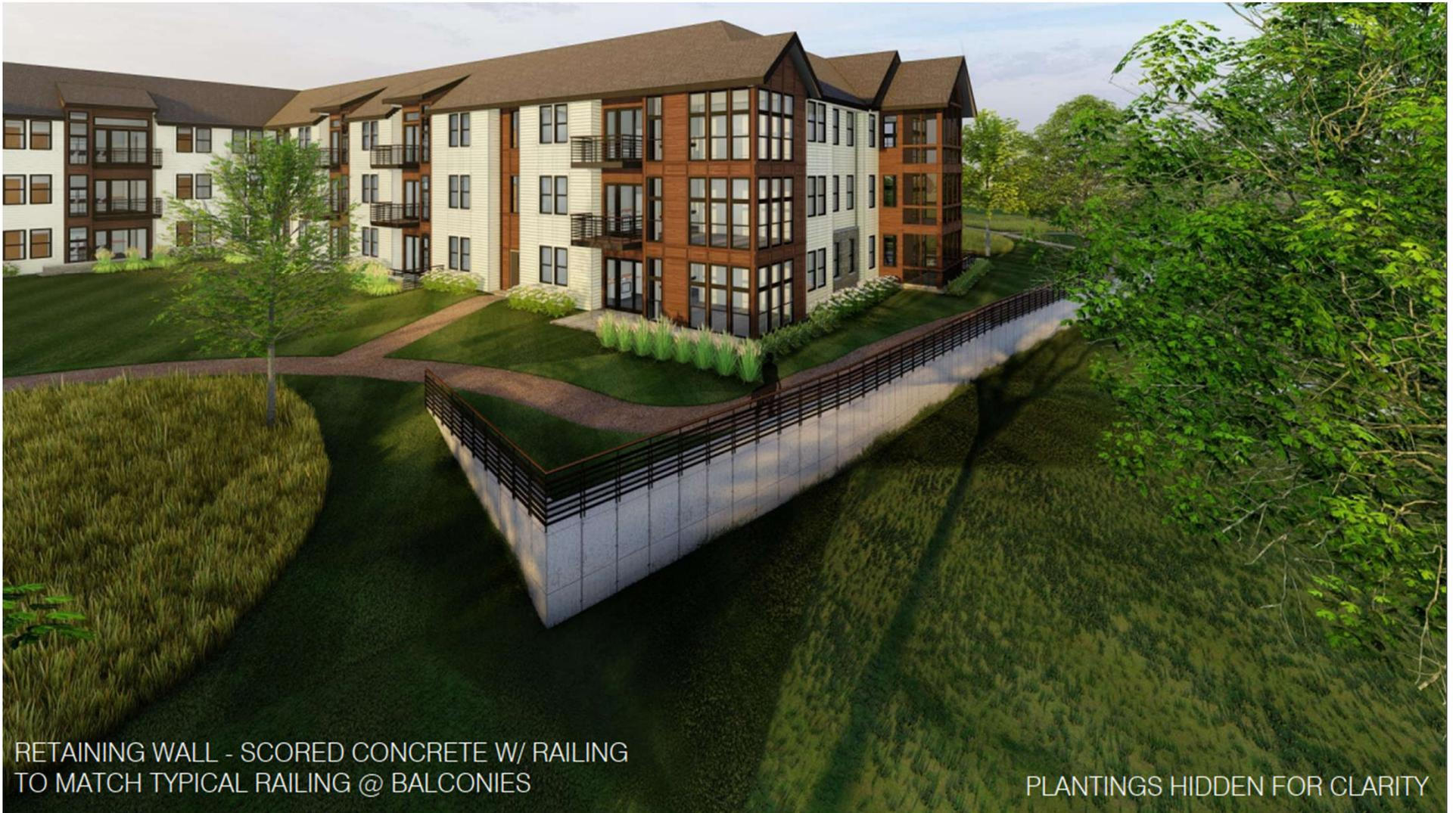
RETAINING WALL - SCORED CONCRETE W/ RAILING
