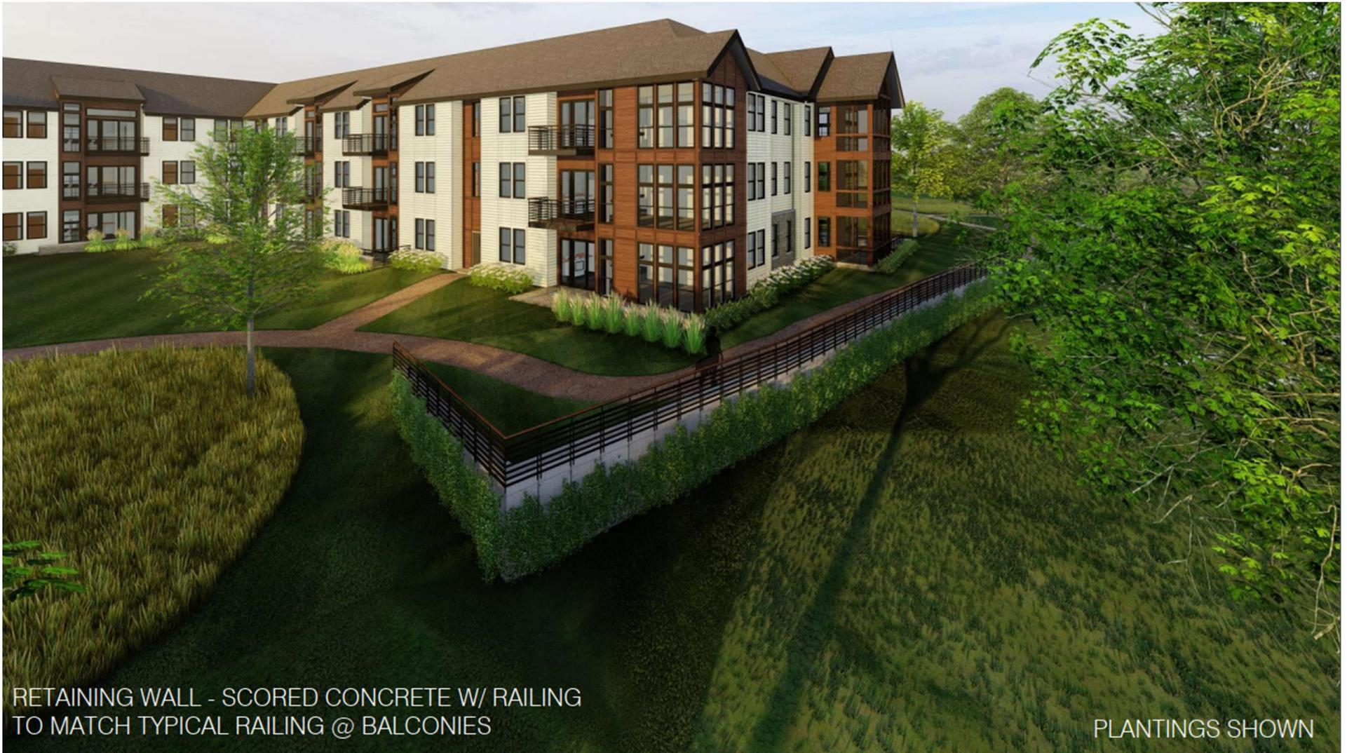
RETAINING WALL - SCORED CONCRETE W/ RAILING
